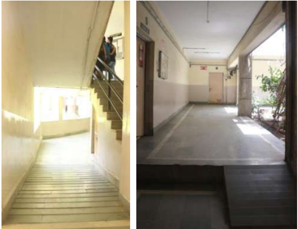
Ramp and Rail
