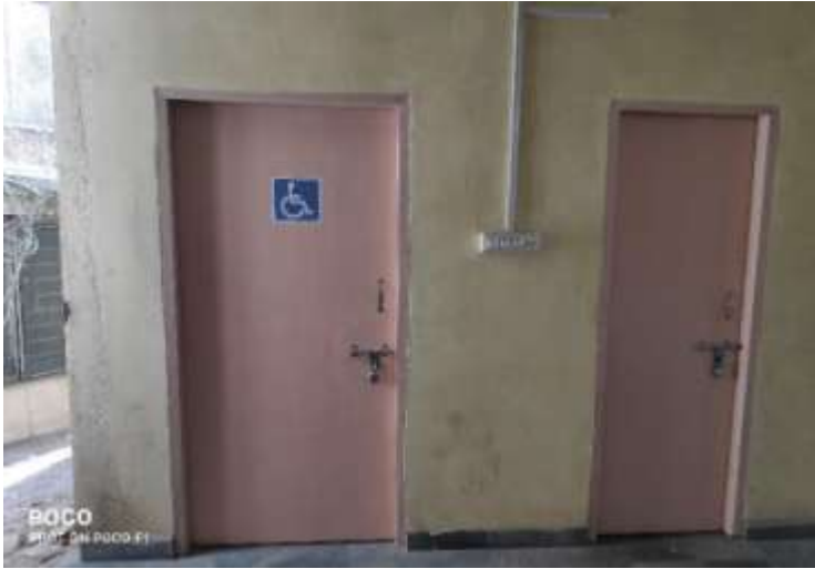
Disabled Friendly Washroom
